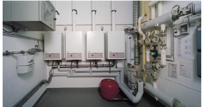
Pressure switch DL safeguards every flue gas route in the cascade
